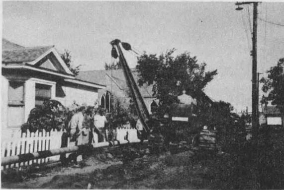
Fig. 1. The cost of corrosion. A 6" gas main no longer serviceable because of leaks, is being replaced by new pipe at left.
