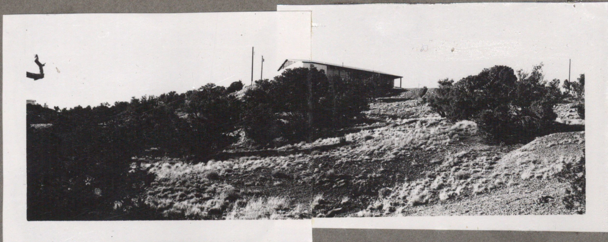
Figure 5. Looking towards the existing building from southeast corner of the site.
