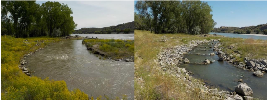
Figure 62. Looking downstream into lower portion of bypass on June 13th (L) and August 20th (R).
