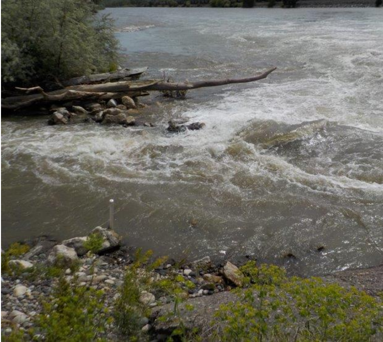
Figure 18. Flow behavior at most upstream end of bypass channel, including wave cresting over upper "weir".
