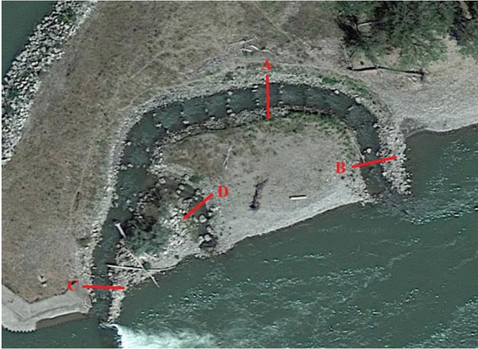
Figure 5. Locations of cross sections used for flow rate determination at the Huntley Diversion nature-like bypass channel (Google Earth, 2020).
