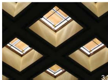
Skylights in Main Sanctuary
