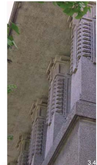
Exterior Concrete Detail
