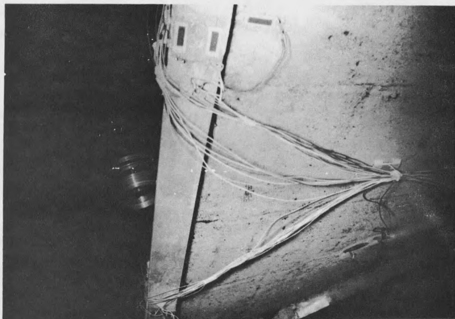
Figure 7. Gages Located On The Underside Of The Structure.
