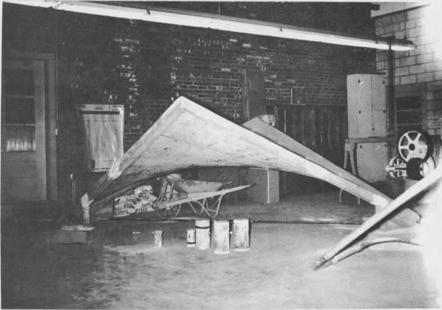
Figure 5. The Finished Shell.
