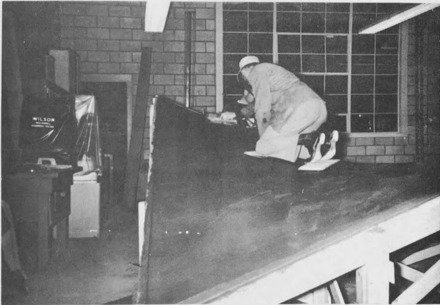
Figure 3. Finishing The Shell Surface.
