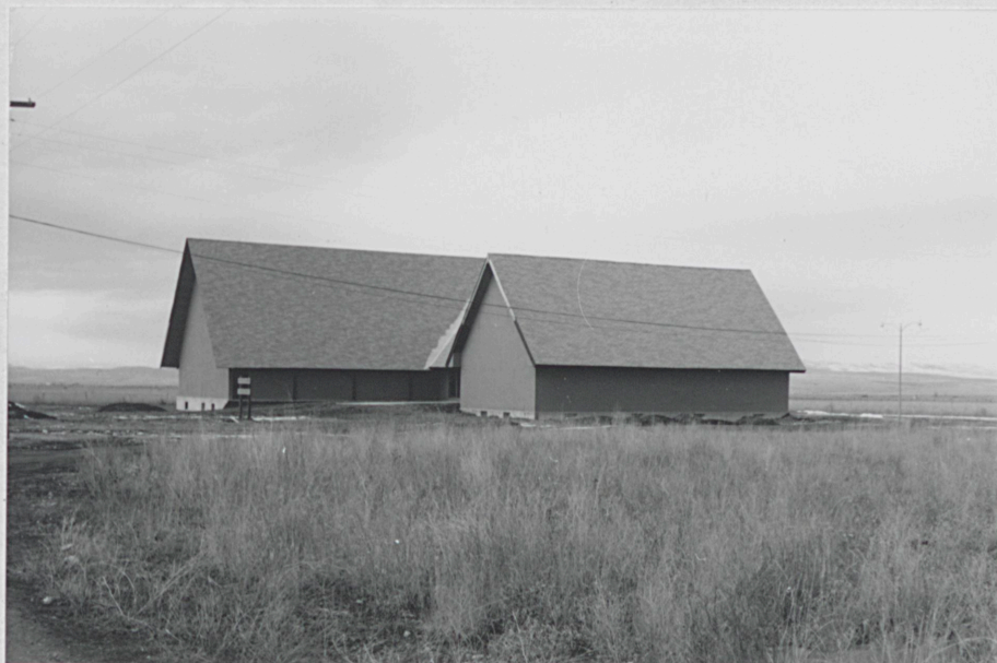
NEW CHURCH, BEING COMPLETED
