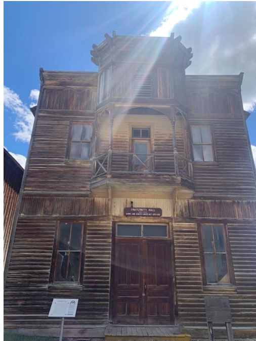
Figure 4. The outside of the Fraternal Hall in Elkhorn, MT
