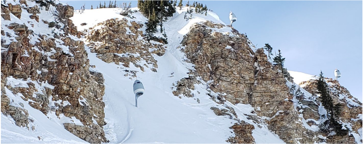
Figure 9 Several operational O'Bellx systems installed at Alta, Utah.
