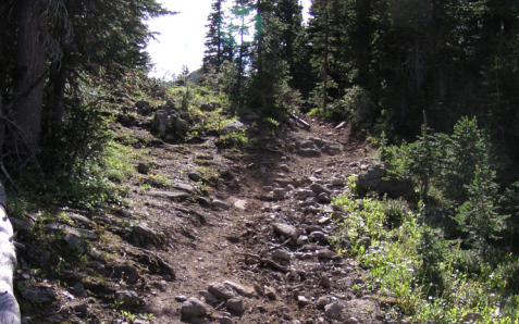
An Emerald Lake user created trail (illegal). Where erosion inevitably becomes impassable, users braid new trails around spreading the destruction. - photo by Phil Knight
