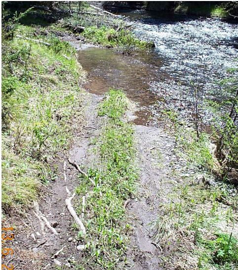
Swan Creek Trail, motorized vehicle erosion of bank, breaching creek results in loss of habitat at site and further down. photo by Phil Knight
