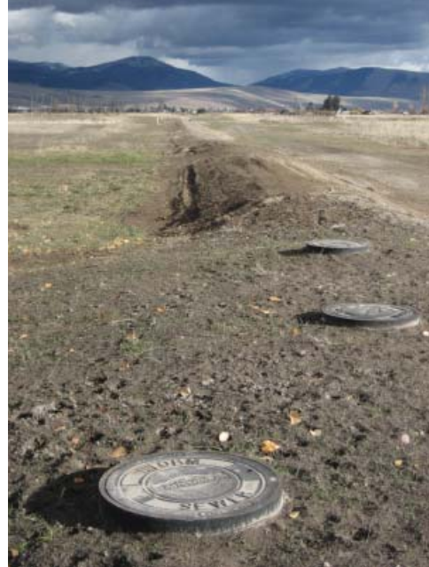
fig. 29 the start of a new subdivision adjacent to the site in prime agricultural soils
