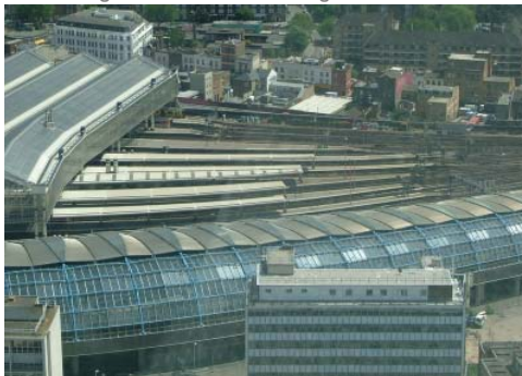
fig. 53 Waterloo aerial of domestic platforms and international trainsheds, London
