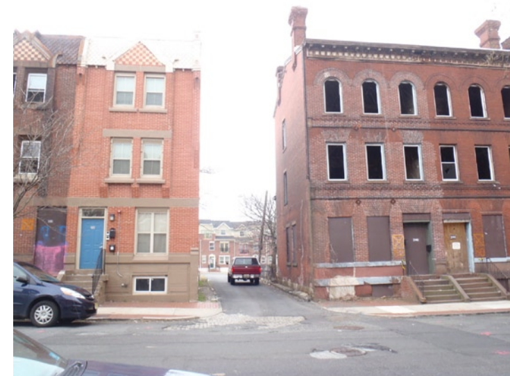
9. Looking west at alley from N. Warren Street
