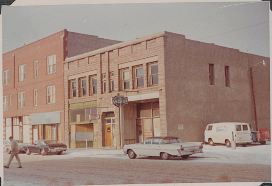
Views of the site from the southeast.
