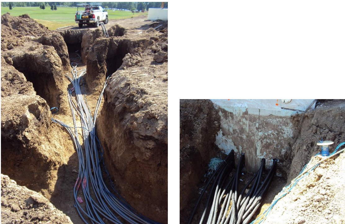
Figure 16. View of the distribution trench and detail of entry to the house through the wall during construction
