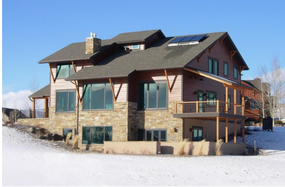
Figure 9. View of the REHAU® Montana ecosmart house
