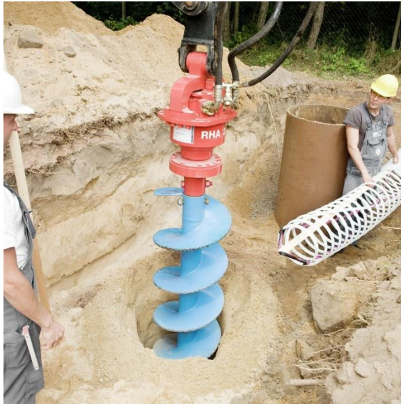
Figure 14. Earth auger creating the borehole for a helix probe. This is one of the key reasons why this type of installation can be a cost-effective alternative to the conventional deep boreholes (Source: www.rehau.com )
