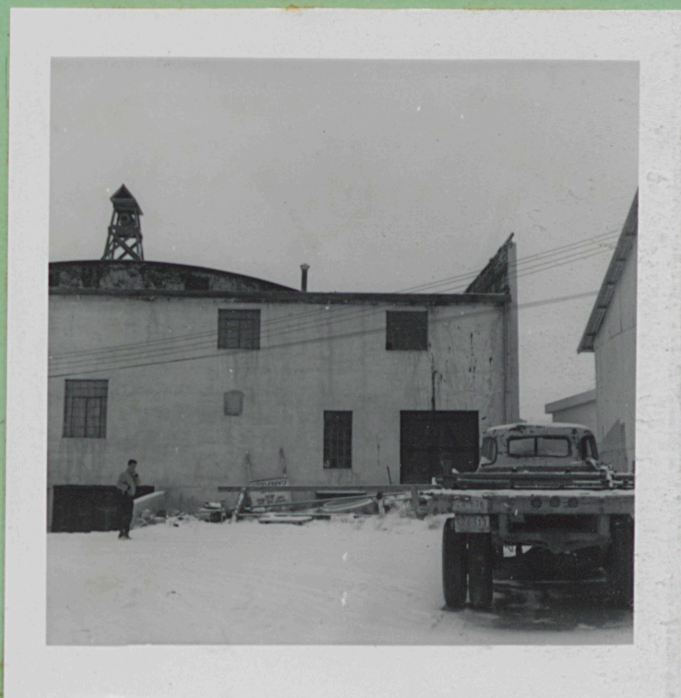
Figure 14. Rear of the Existing Building
