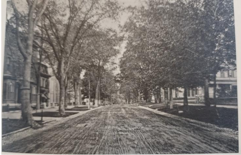
Figure 3.8. This section of State Street in Portland, Maine, 1901, included smoothly paved sidewalks, curbstones, cobblestone gutters, and a dirty roadbed. Image published in Souvenir of Portland, Maine , viewed at the Brown Research Library, Maine Historical Society.
