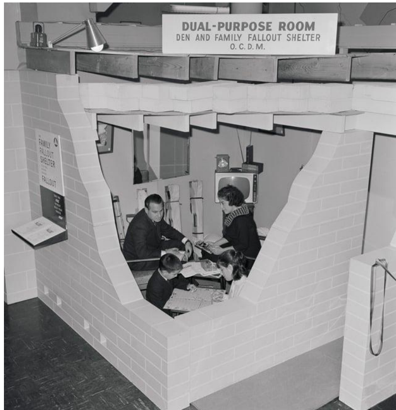
Figure 5.10. A demonstration basement fallout shelter prepared by the Office of Civil Defense Mobilization amounted to a second foundation wall of concrete blocks and cement mortar that connected to the existing foundation walls. The image gives a sense of why most American homeowners with a
