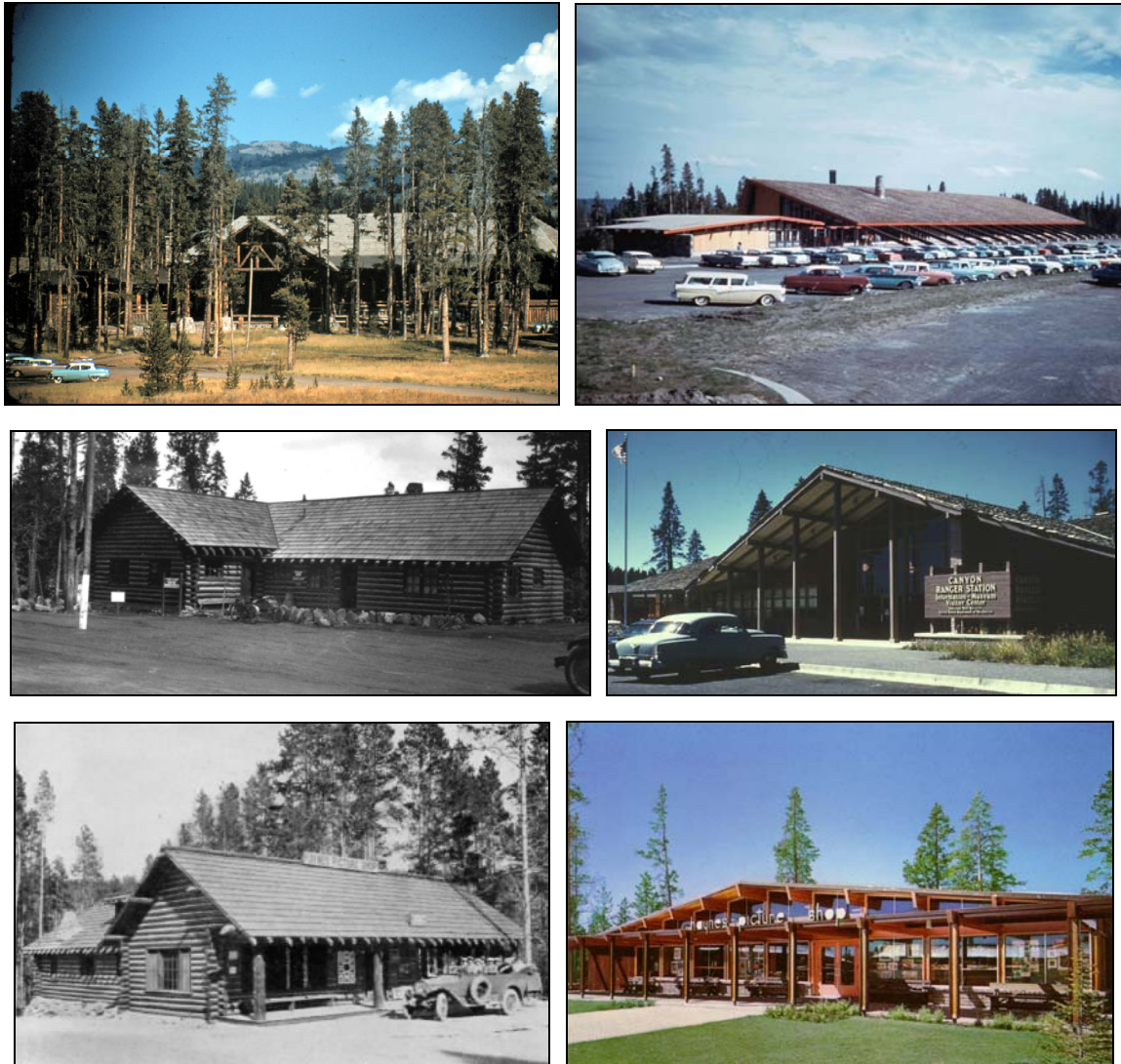
Figure 137: Exterior Cultural Environment Rephotography Pairs: Top left—Old Canyon Lodge, early 1950s by Stempel (Stempel Collection); Top right—New Canyon Lodge at Canyon Village, 1957 by Haynes (Whittlesey Collection); Middle left—Canyon Ranger Station (Yellowstone Museum Collection); Middle right—Canyon Ranger Station/Visitor Center, 1960 by Haynes (Whittlesey Collection); Bottom left—Haynes Picture Shop, 1924 by Haynes (Goss Collection); Bottom right—Haynes Picture Shop at Canyon Village (Francis Collection)
