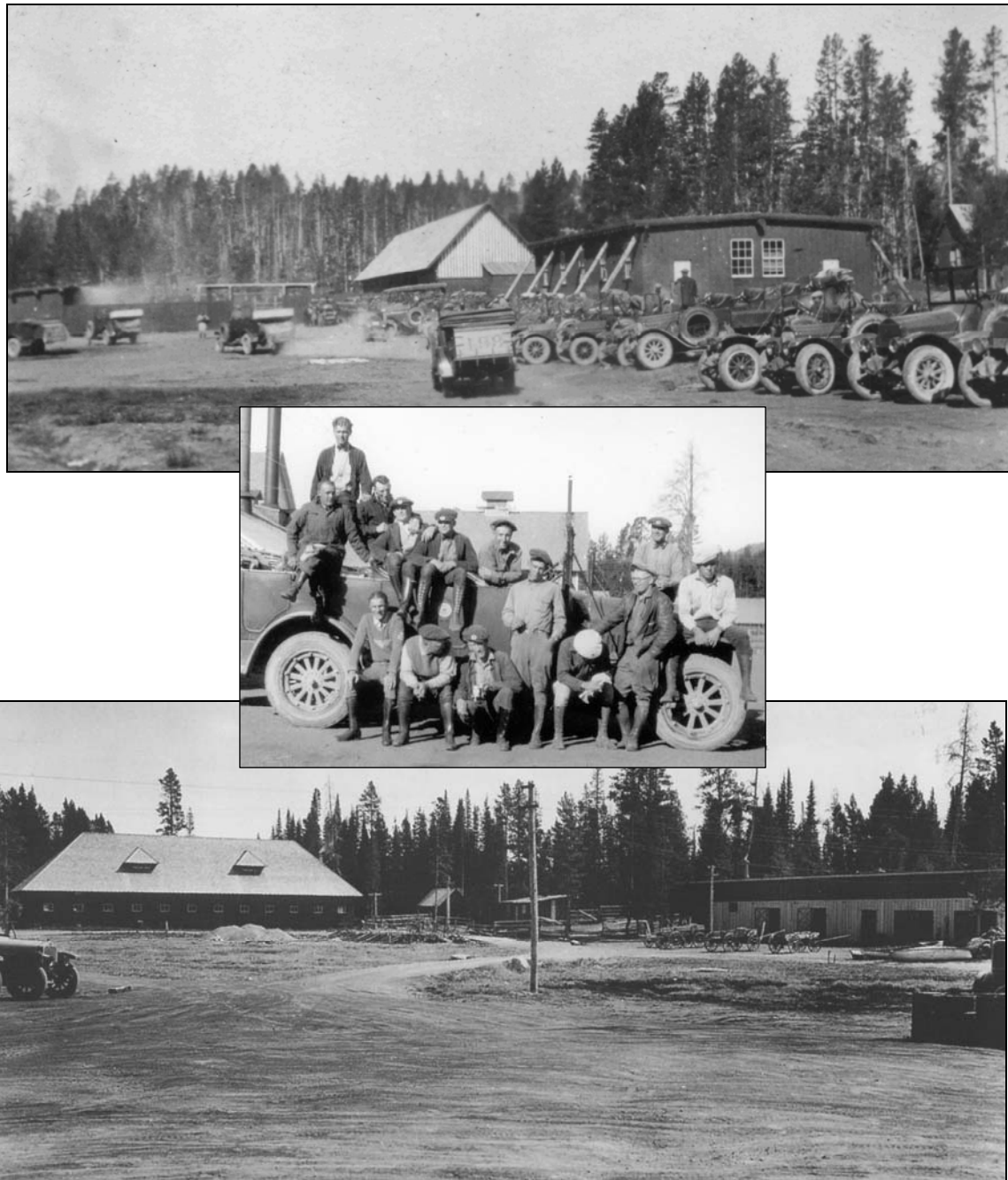
Figure 75: Canyon Bus Complex: Top—Reamer’s Coach Shed (pitched roof) incorporated into the “Bull Pen,” and new Repair Shop, circa 1924, west view (Yellowstone Photo Collection); Middle—Park bus drivers (possibly Cody Drivers) shown probably behind Lake Hotel, 1922 or 1923, including Gary Cooper standing on bus at left and Ralph Bush, Sr. sitting at right in white shirt (Bush Collection—identification source is Bush email 01/16/06); Bottom—Reamer’s Hay Shed converted to the Cody Bunkhouse with hotel horse corrals and stables nearby, 1929, east view (Quinn 2004a)
