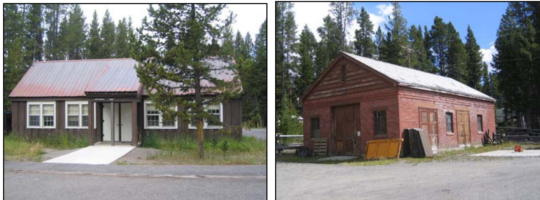
Figure 97: Canyon Utility Area Pre-War Structures: Left—Mess House with quarters (Building 323) constructed 1940; Right—Powerhouse (Building 322) constructed in 1941 (author photos, 2005)
