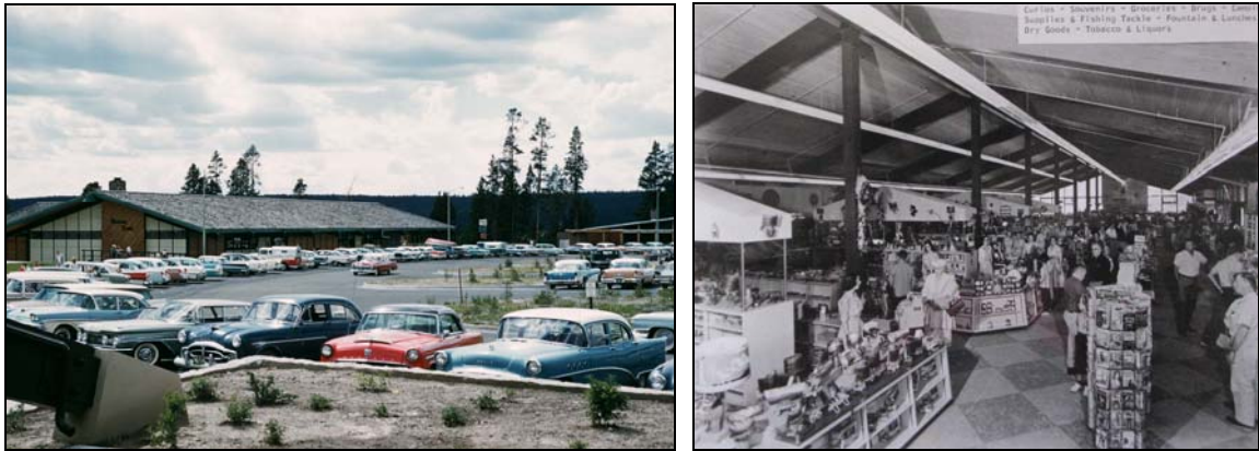
Figure 121: Hamilton Store at Canyon Village: Left—Parking lot and store exterior (Whittlesey Collection); Right—Store interior (YPSS Archives)
