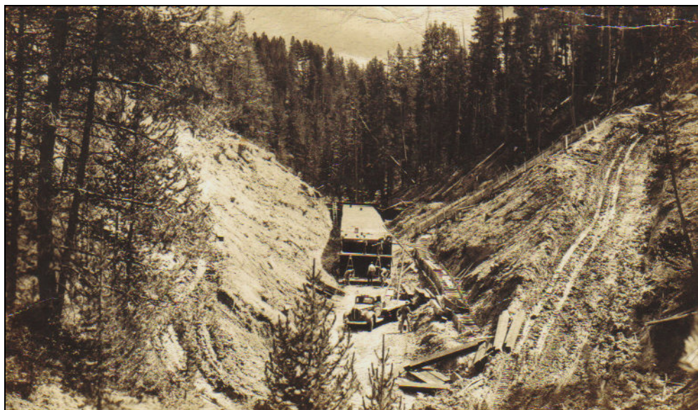
Figure 98: Grand Loop Road Bypass at Canyon: Top—1941 master plan (Yellowstone Archives); Bottom—Cascade Creek box culvert before infilling for Grand Loop Road bypass, 1941 (Morse Collection)
