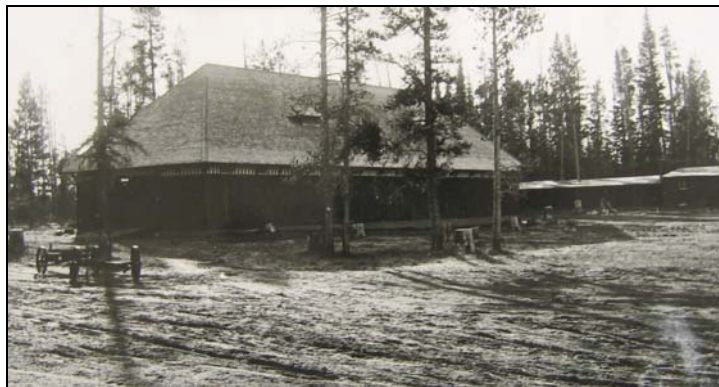
Figure 42: Reamer-Designed Buildings at Canyon Transportation Complex: Top—Coach shed (Yellowstone Museum Collection); Middle—Coach stables (Yellowstone Museum Collection); Bottom—Hay barn with corrals in background (Yellowstone Museum Collection)
