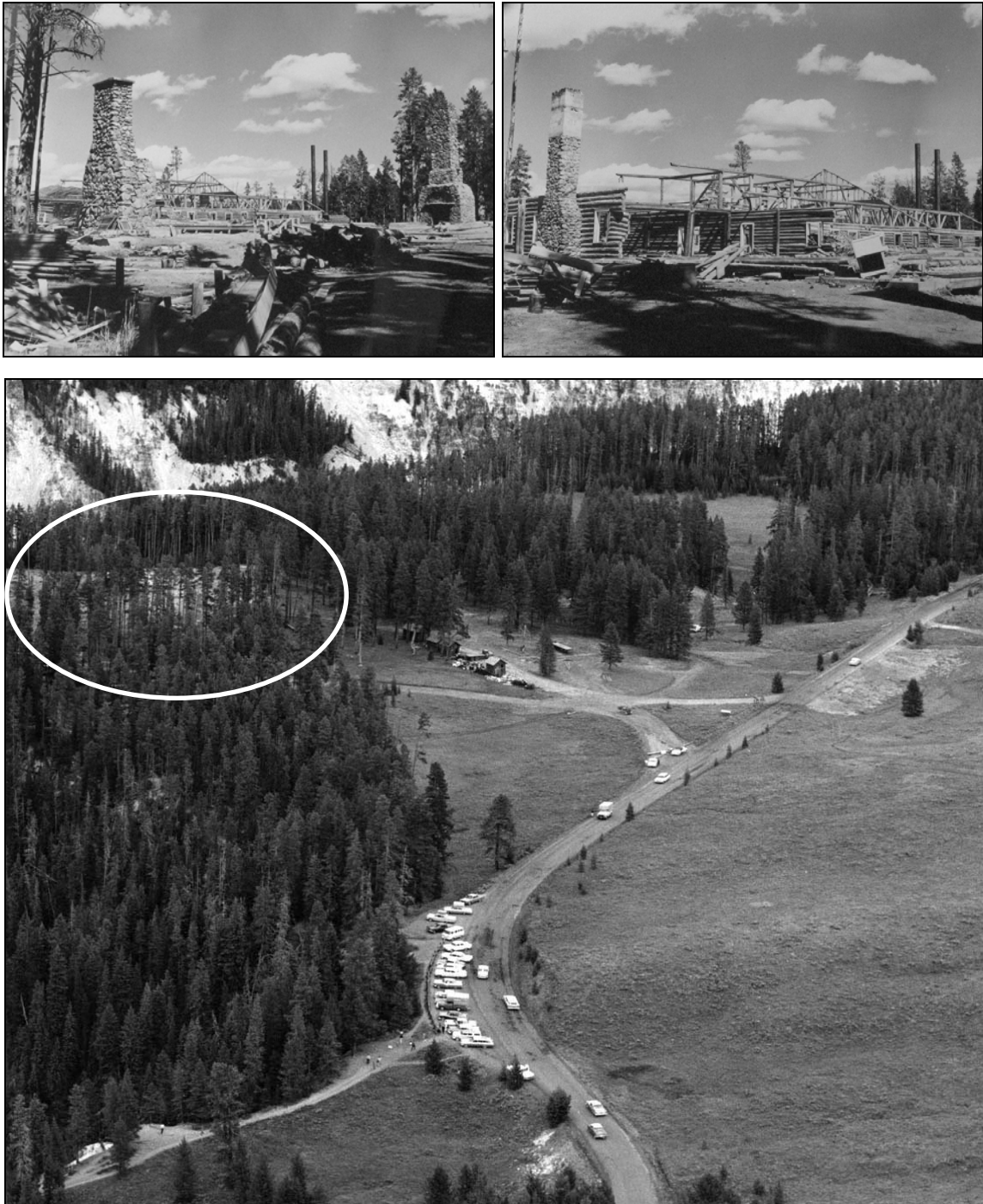
Figure 127: Canyon Lodge Dismantling: Top left—Willson's 1925 lobby west and east fireplaces still standing; Top right—Dismantling of original Shaw and Powell dining room and 1921-1923 kitchen addition (Yellowstone Museum Collection); Bottom—Cabin removal work underway, July 1959 (lodge site circled), with tourists parked at Upper Falls eastern overlook parking area (Yellowstone Photo Collection)
