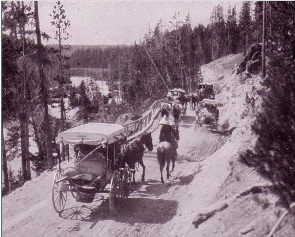
Figure 21: Sagebrushers Meet Stagecoaches along the West Rim: Chittenden Bridge in distance c1913. Probably south of Canyon Bridge (Francis Collection)
