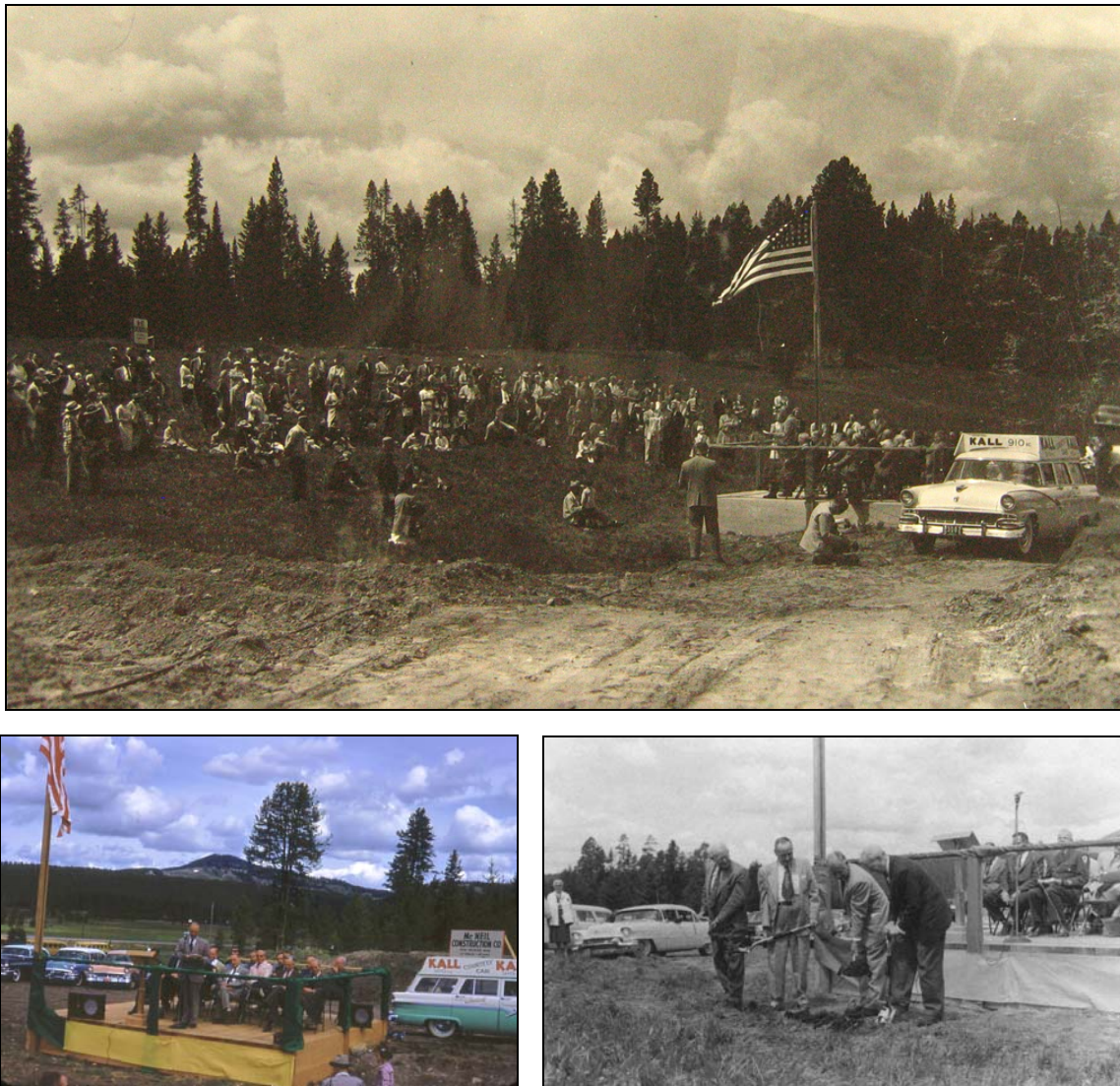
Figure 116: Ground Breaking Ceremony, June 25, 1956: Top—Ceremony setting (Yellowstone Museum Collection); Bottom left—Invited guests and Wirth delivering remarks (Whittlesey Collection); Bottom right—Breaking ground, left to right, Haynes, Hamilton, Wirth, and Nichols (Barringer 2002)
