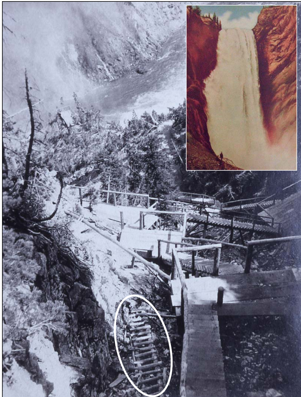
Figure 48: Government-Built Uncle Tom's Trail Infrastructure: New stairway with terminal viewing platform built in 1905-1906 over Uncle Tom's Trail, photo by Al Noyes, 1906. One of Uncle Tom's ladders circled (Yellowstone Photo Collection); Inset—1911 infrastructure at the west end of Uncle Tom's Trail (Yellowstone Library—Northern Pacific Railroad brochure)
