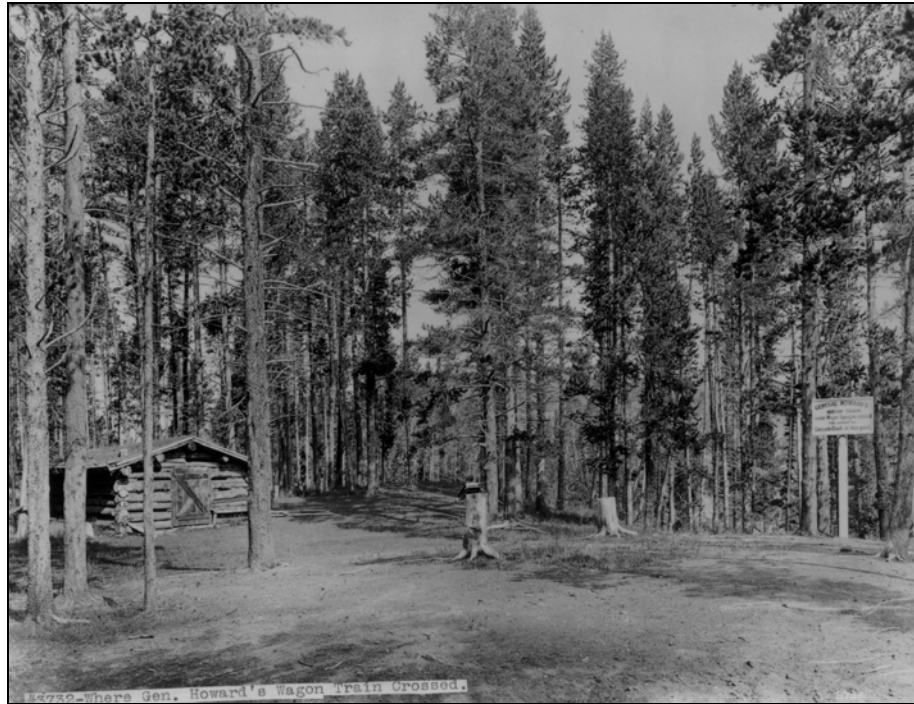
Figure 28: West Rim Road at Cascade Creek. Sign commemorating the route of Spurgin's wagon train. Origin and function of cabin unknown, also shown in Figure 25 (Library of Congress)
