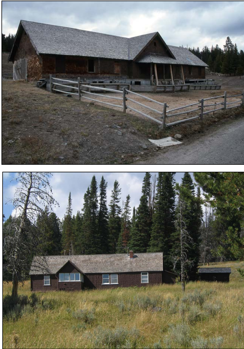
Figure 131: Canyon Hotel Structures Retained: Top—Men's Dormitory Converted to Hay Barn, by Peaco, 1992 (Yellowstone Photo Collection); Bottom—Winterkeeper's quarters, 2005 (author photo)
