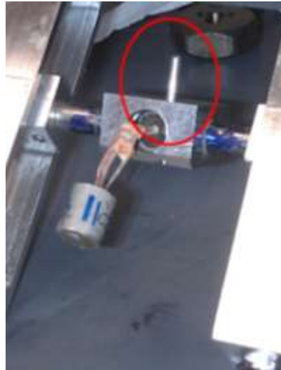
[Figure 9: Locking Pin] Pin in red circle used to keep pot from sliding back out of fixture.
