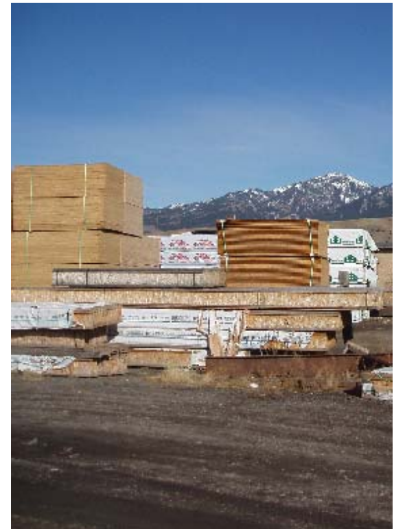
Trash from packaging and scrap material litter the site and pavement covers most developed areas
