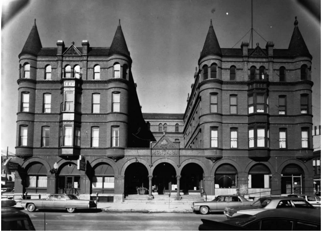
Figure 38. Montana Hotel, ca. 1971. (Library of Congress American Memory Project)
