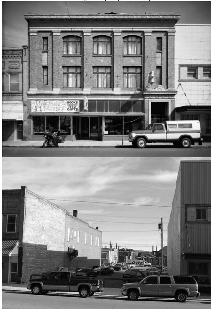
Figure 57. Beneficial Life building on Main Street in 1981 (top) and 2004 (bottom). (top, Library of Congress American Memory Project; bottom, Author's collection)
