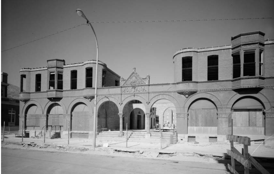
Figure 50. Montana Hotel under demolition, 1979. (Library of Congress American Memory Project)
