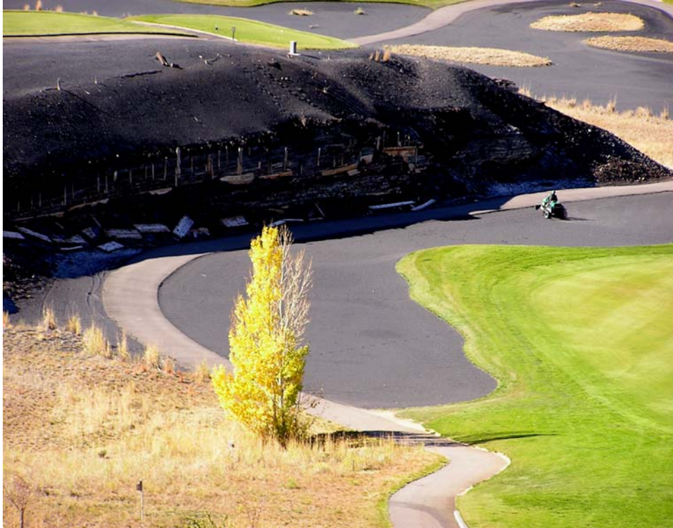
Figure 64. Slag traps at the Old Works golf course in Anaconda, 2004. (Author's collection)
