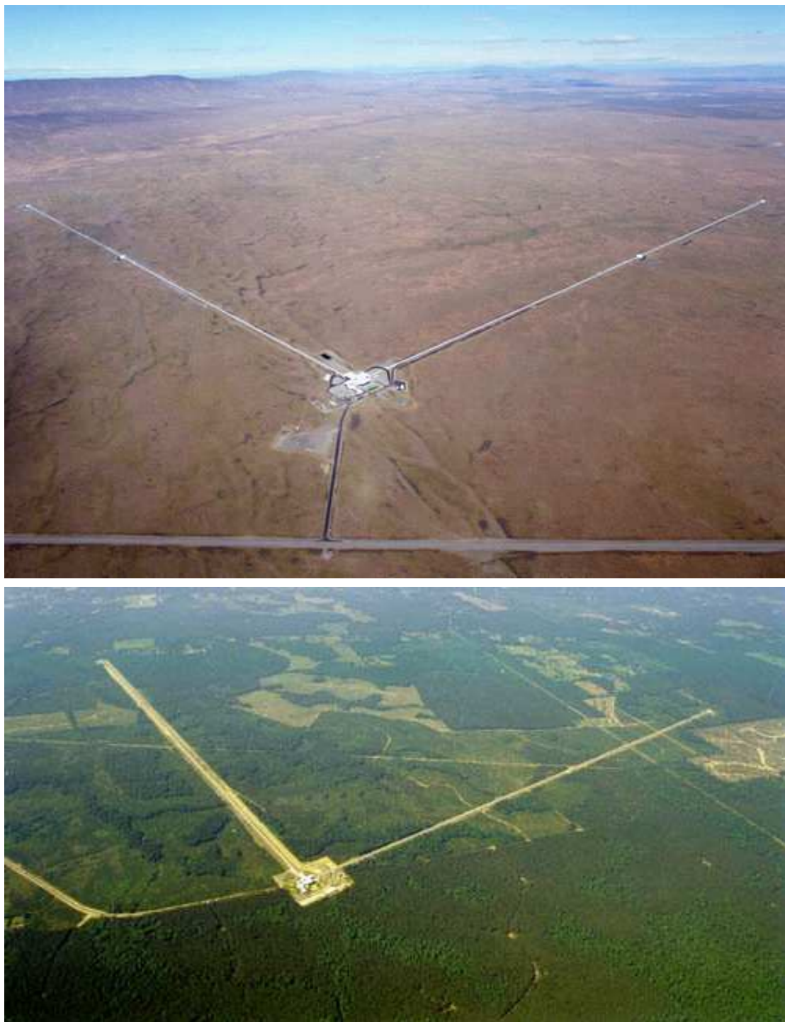
Figure 1.2: Aerial photographs of the LIGO facilities in Washington (top) and Louisiana (bottom).
