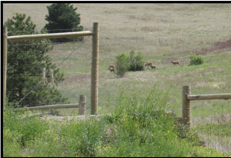
Figure 5. A jump-out as seen from the road corridor.
