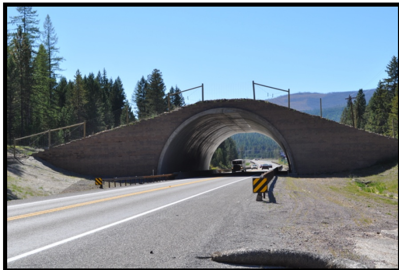
Figure 3. Wildlife crossing structures, including a medium culvert, large culvert, bridge and wildlife overpass.
