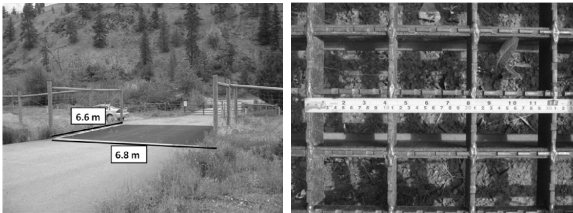
Figure 7. Wildlife guard and grate dimension.
