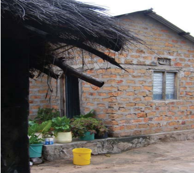
Fig 2.13 A traditional house against a new 'modern' well built brick dwelling. The traditional dwelling has adequate ventilation, the newer one does not
