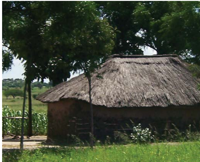
Fig 2.16 Traditional Sukuma dwelling - mud plaster over adobe and thatch
