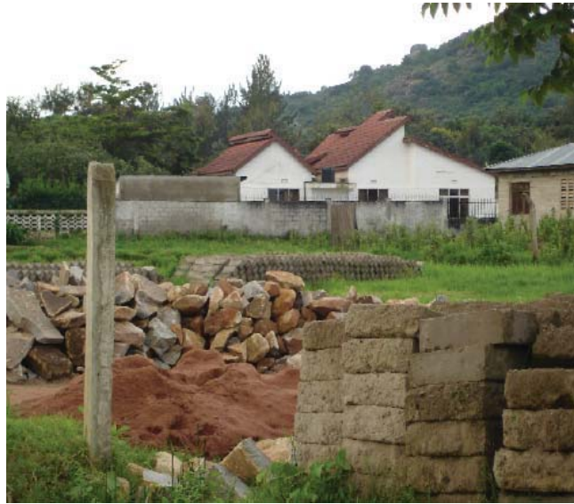
Fig 4.9 a pile of local and site-made materials sits on a future building site
