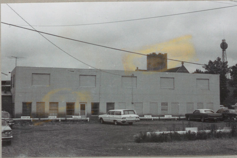
Rear of existing building and its parking facilities.
