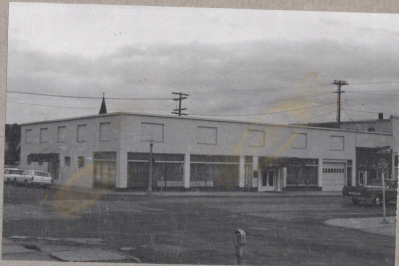
Existing building, main entrance from across South Wilson and Babcock intersection.
