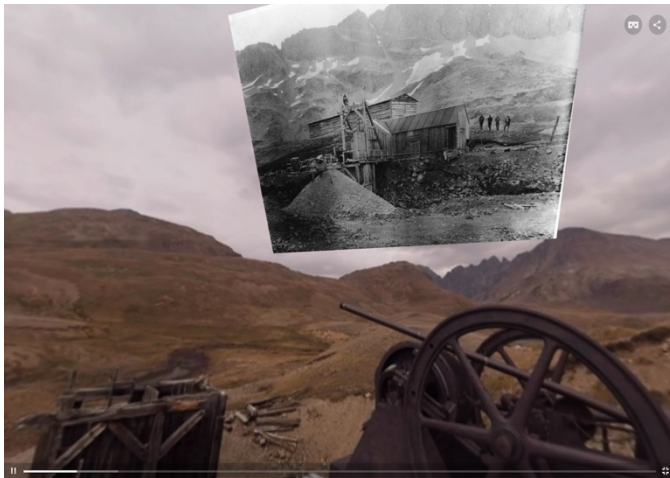
Figure 11: Locations such as Goose Lake are within the wilderness boundary of the Absaroka-Beartooth Wilderness. Accessibility to this location requires visitors to own or rent ATVs and hike up to the location. A historical photo shows what the abandoned Copper King Mine once looked like at the turn of the 20 th century. Image from: A Road Through the Wild .
