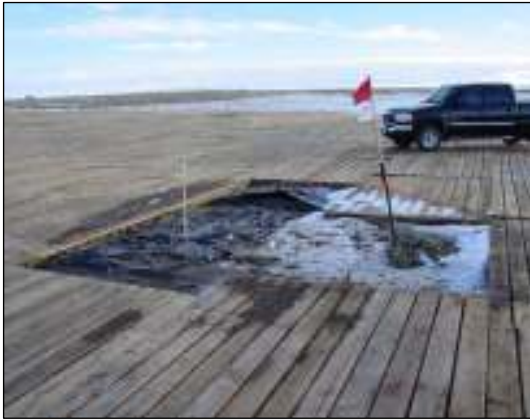
Figure 2. View of a drill pad constructed with oak mats.
