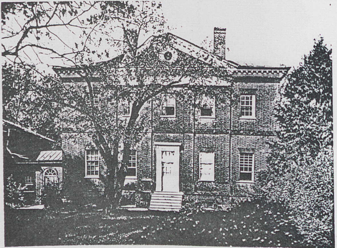
Garden Elevation, Harwood House, Annapolis, MD.
