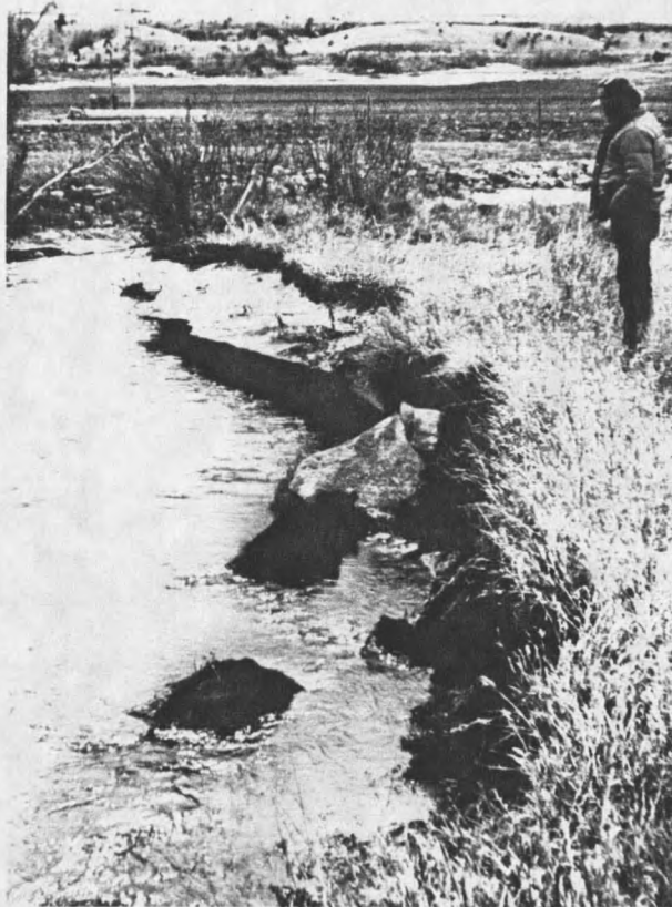
Figure 30. Erosion due to ice along outside bend of Deep Creek during spring thaw, March 1989.
