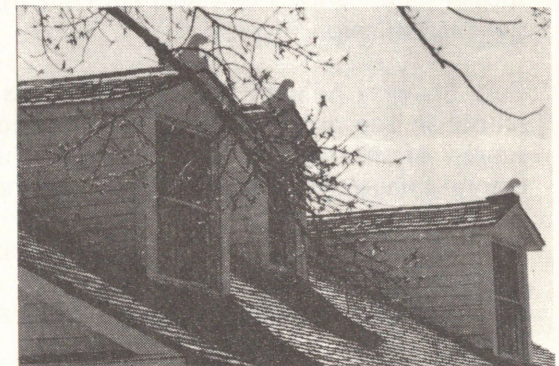
Refined dormers on Officer's Quarters
