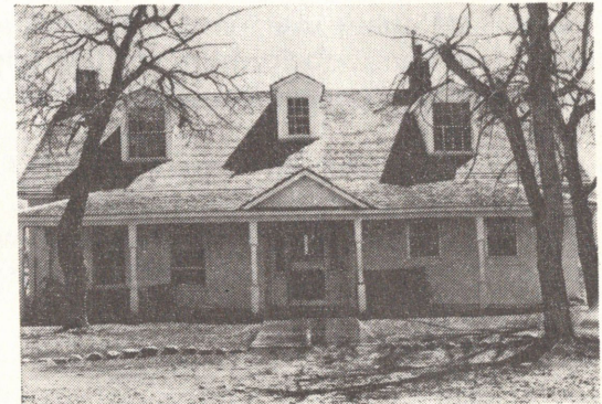
Officer's Quarters at Fort Shaw
