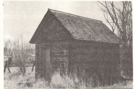
Storehouse at Fort Shaw
