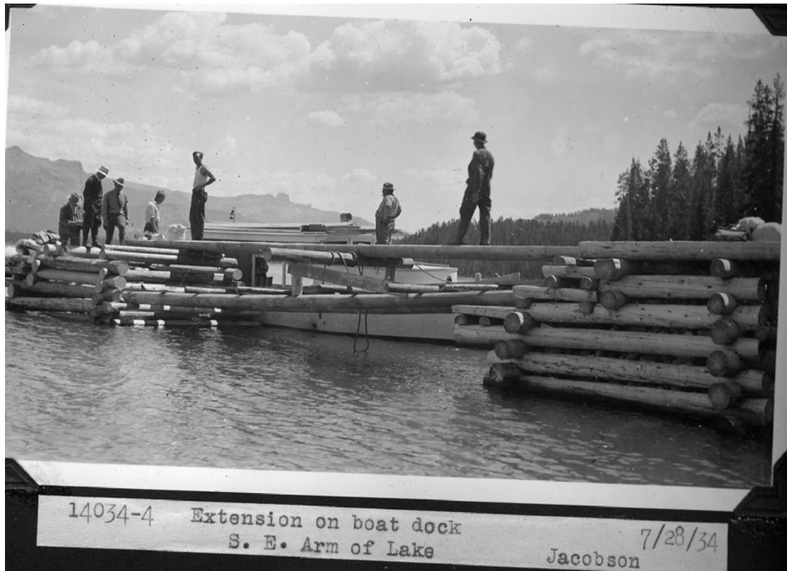
Figure 77. Boat Dock at the Southeast Arm of Yellowstone Lake, 1934 As motor boats became a more common sight on Yellowstone Lake, the National Park Service and concessionaires focused more of their attentions on the southern realms of the lake. This boat dock was located in the Southeast Arm of the lake near Clear Creek. [Courtesy of Yellowstone Park Photo Archives.]
