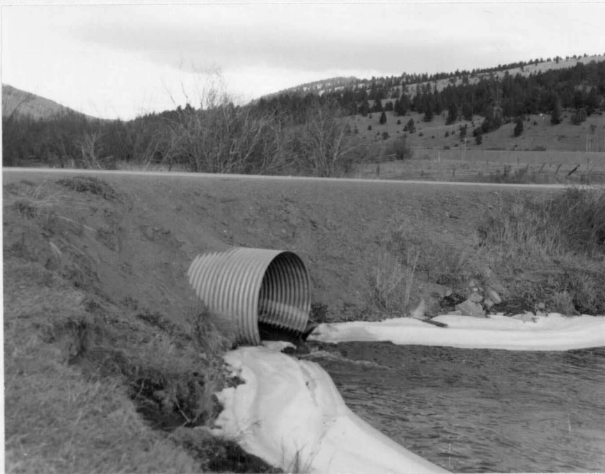
Figure 4 - Photo of culvert at sampling station zero.
