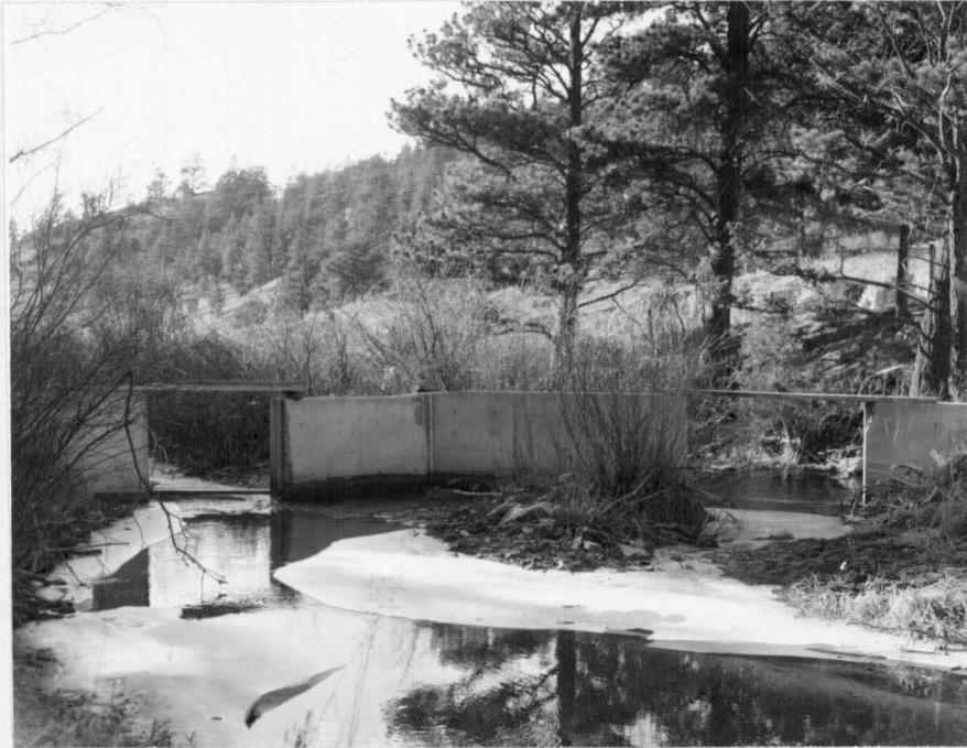
Figure 6 - Photo of concrete control structure located at station one.
