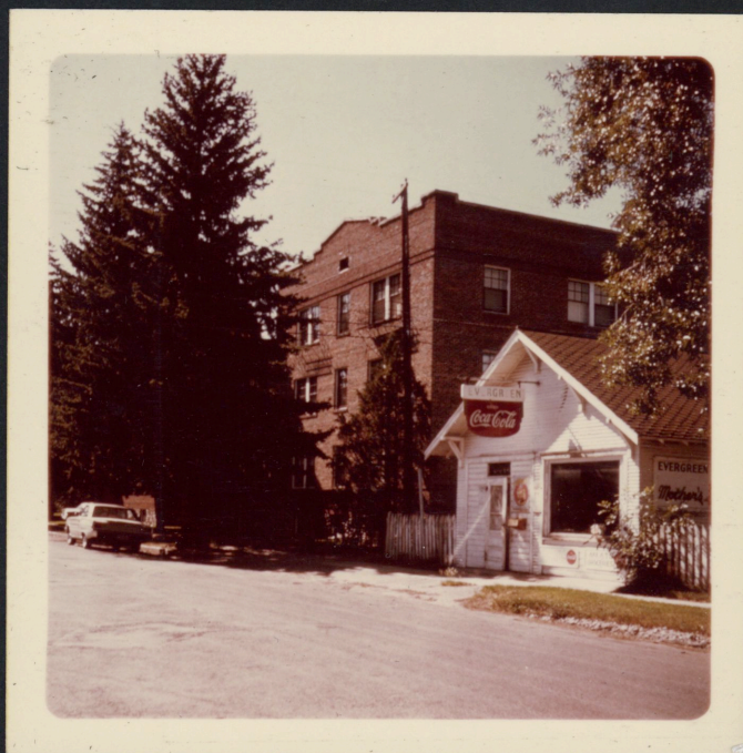
Figure 2. Evergreen Apartments (front view)
