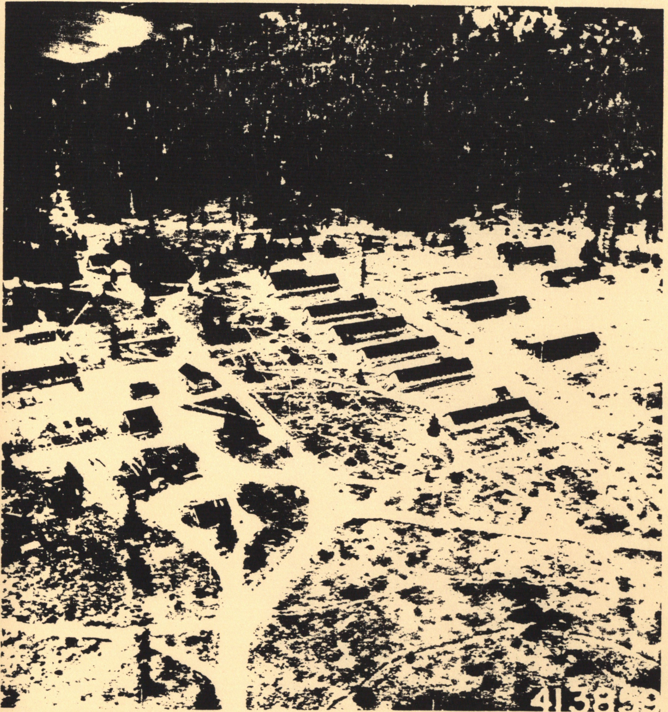
Aerial view of the CCC camp on Stoney Creek west of Missoula, Montana.
