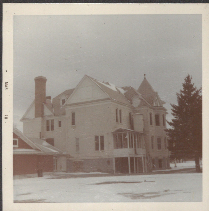
ADMINISTRATION BUILDING LOOKING TO THE SOUTH-EAST
