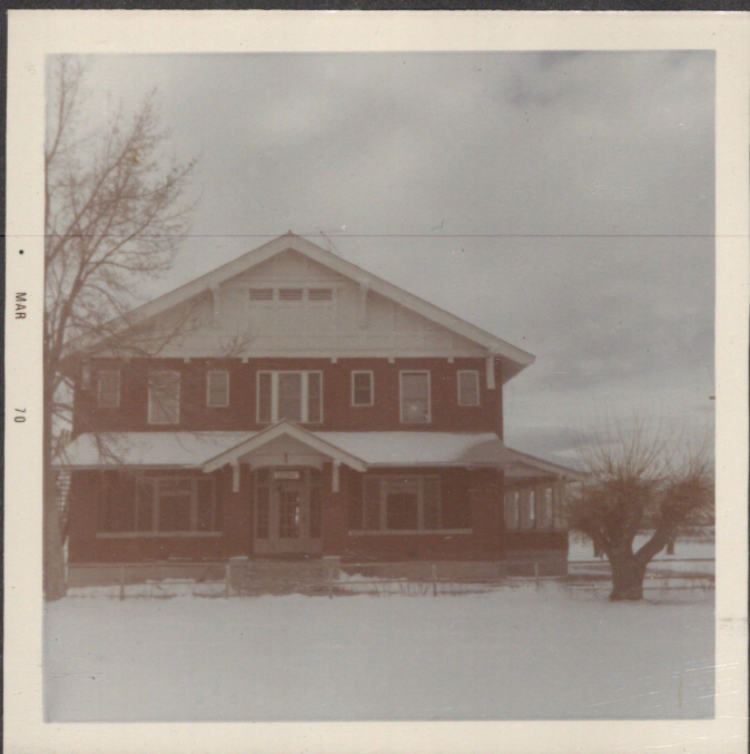
RIVERSIDE COTTAGE LOOKING TO THE NORTH
