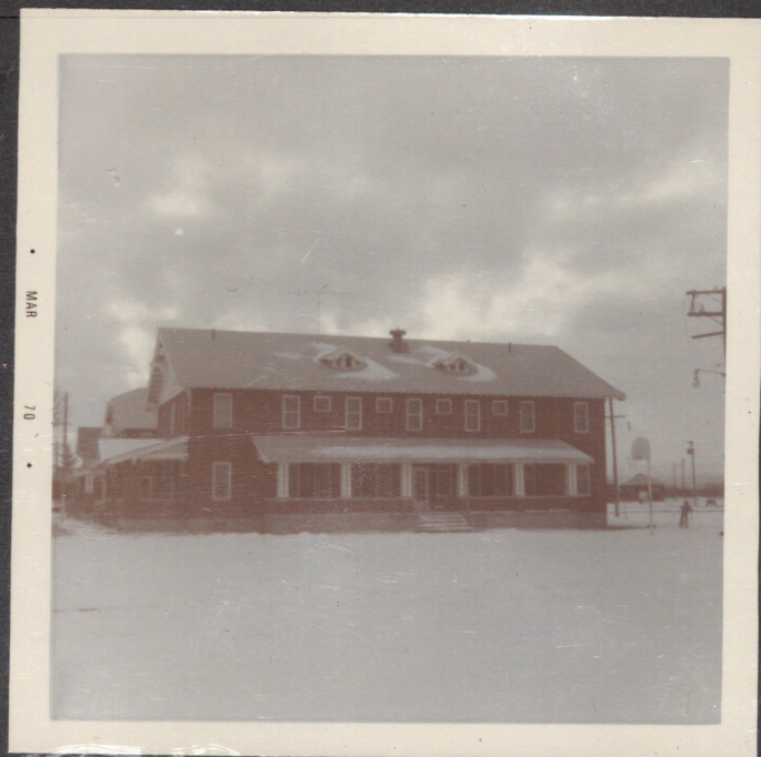
RIVERSIDE COTTAGE LOOKING TO THE WEST
