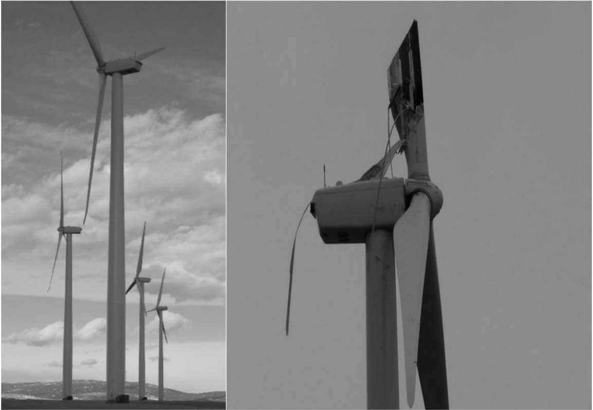
Figure 2: Typical wind turbine (left), with a blade failure (right).
