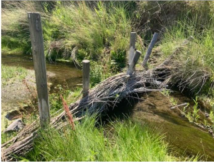
Figure 2. Typical BDA restoration design. Photo by Allison Law.
