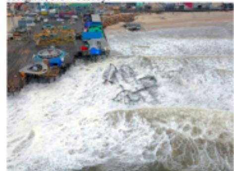
Figure 3.6 B. Coastal Storm Surge Damaged Casino Pier during Hurricane Sandy in Seaside Heights, New Jersey.
