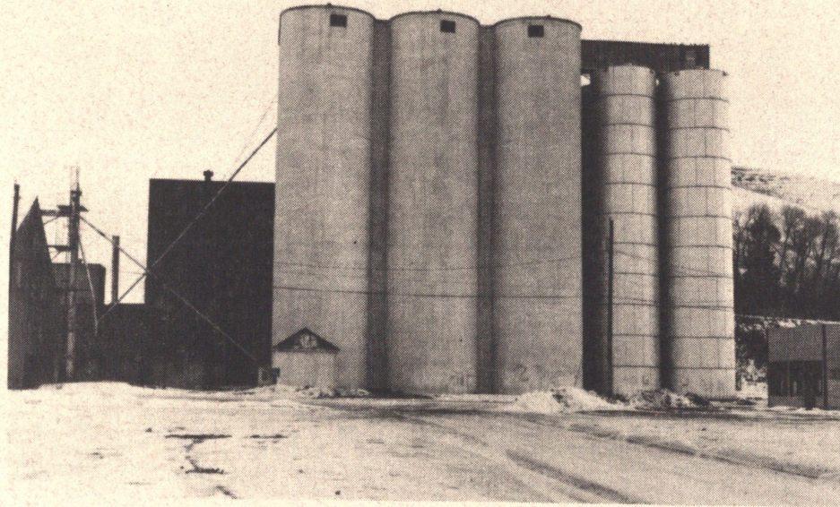
19. Grain storage tanks, storage building (on left) and mill building (looking East).
