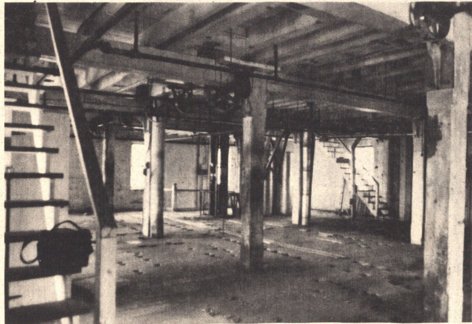
15. View to Northeast corner of mill building, third floor. Notice holes in floor and ceiling where drive belts once ran between floors.
