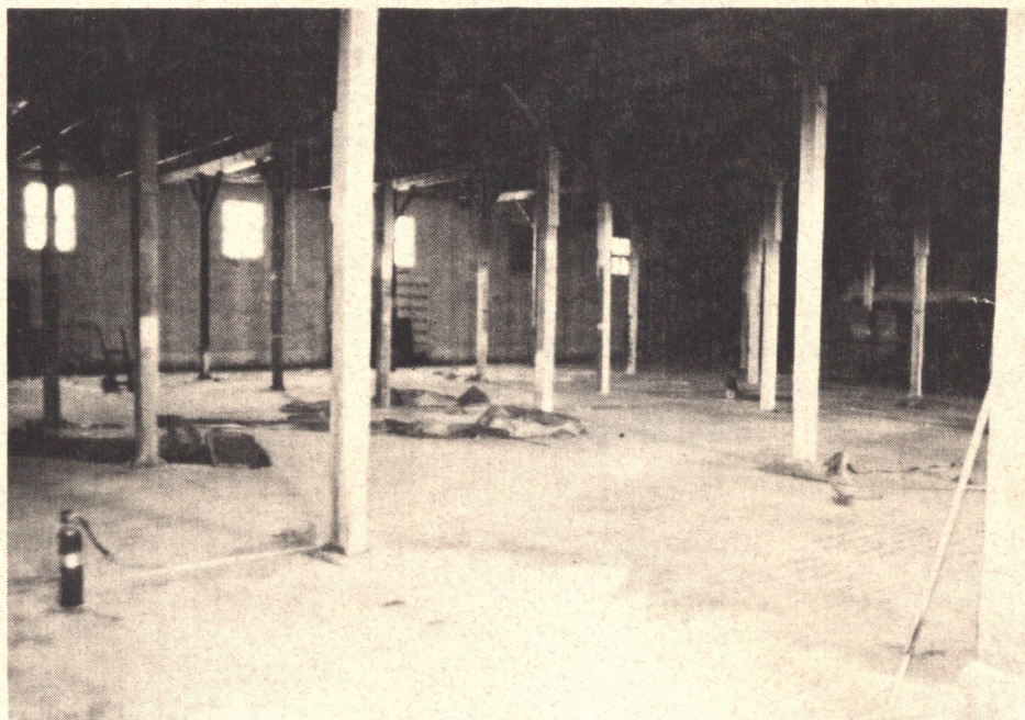
18. Warehouse from first floor looking Southeast.
