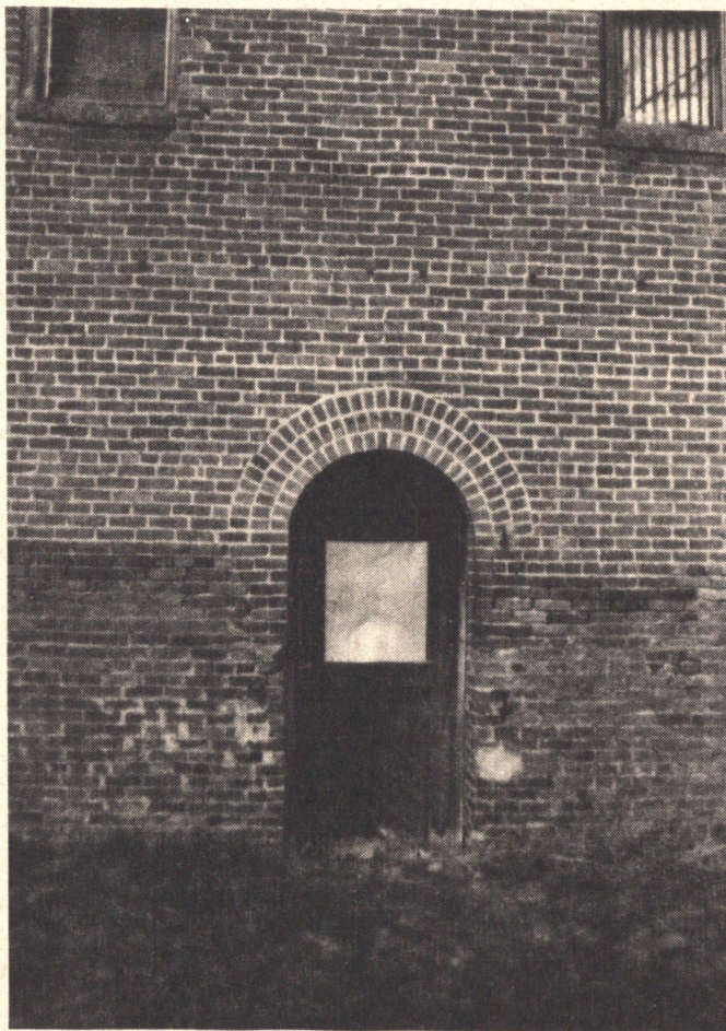
1. South side of the old shop building.
