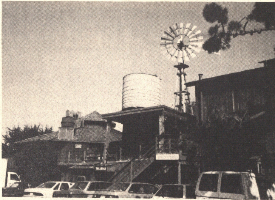
27. View from parking lot showing outbuildings and water tower.
