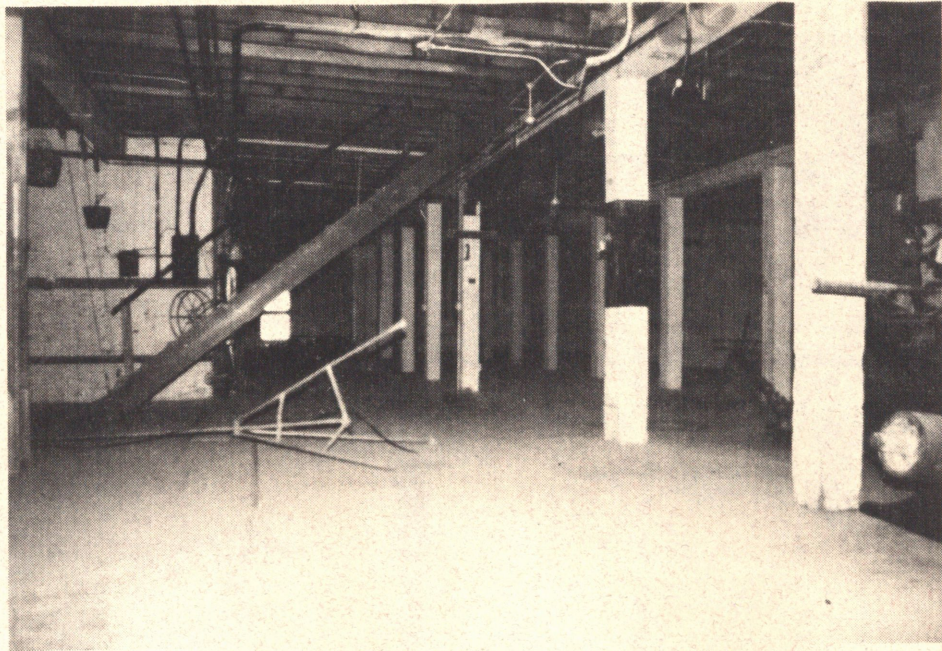
13. Second floor of intermediate space between mill and warehouse (looking South).
