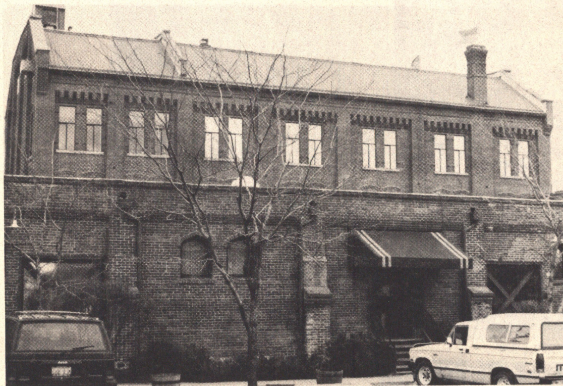
26. Exterior view looking at West facade.
