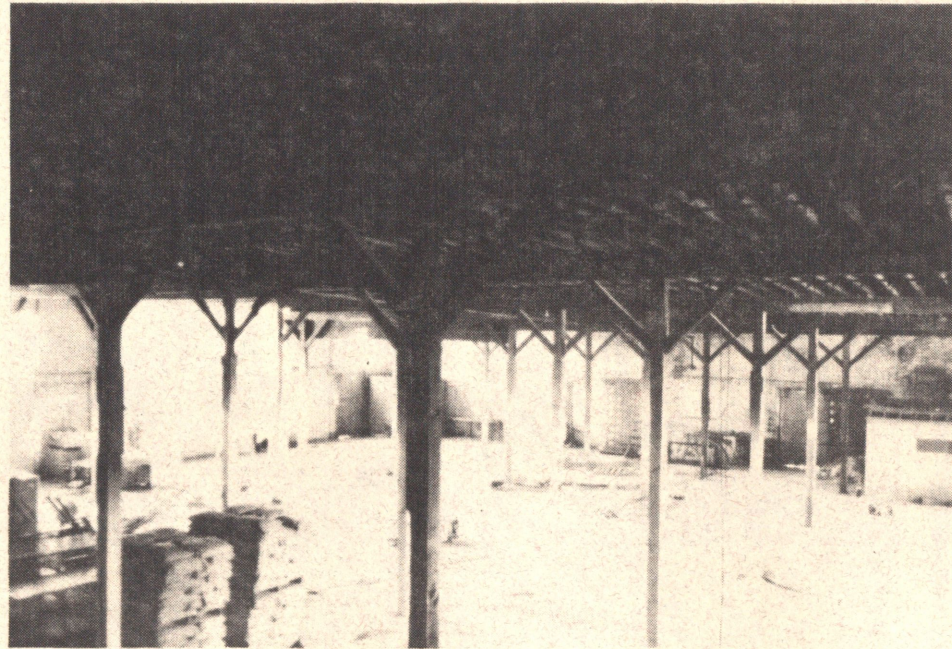
14. View of warehouse from second level Southeast corner.
