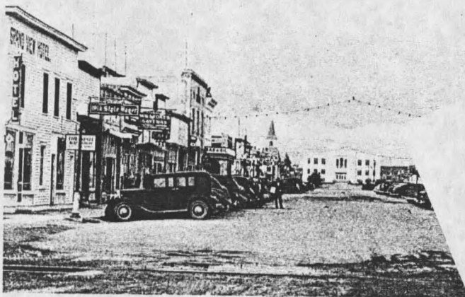
Main Street looking north. Late 1930's
