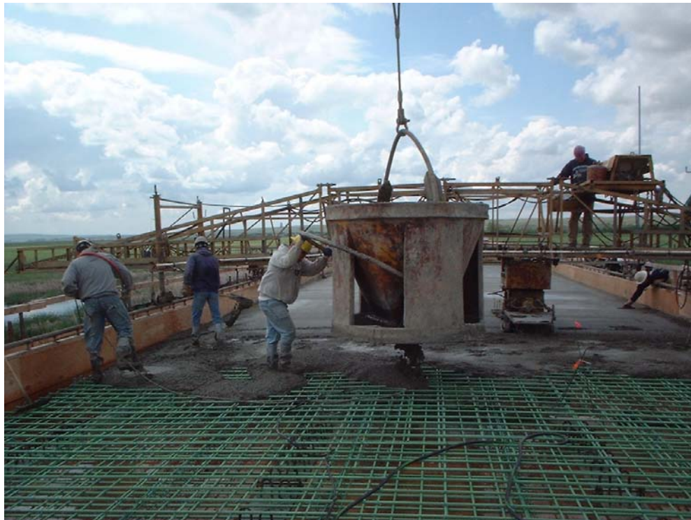
Figure 33. Placing the Deck Concrete
