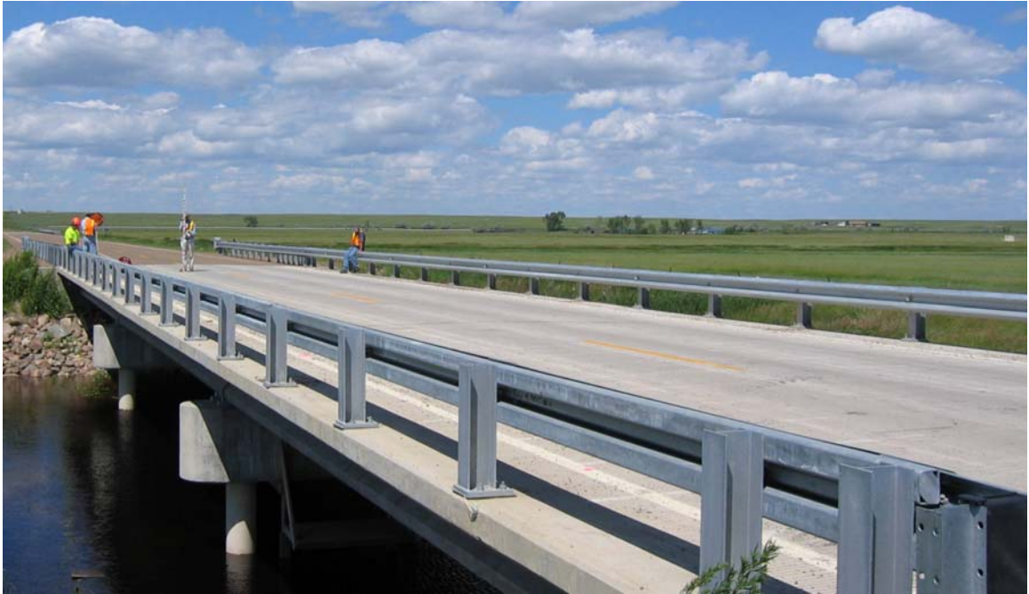
Figure 27. Completed Bridge Deck
