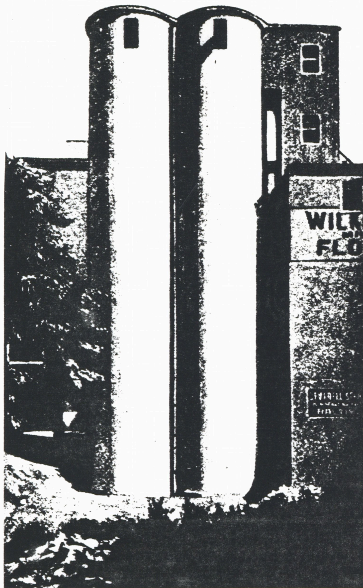
10. Grain elevator from Le Corbusier's "Toward a New Architecture."
