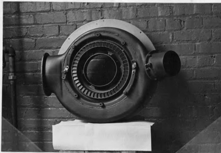
Fig.34-Turbine Nozzle Box
