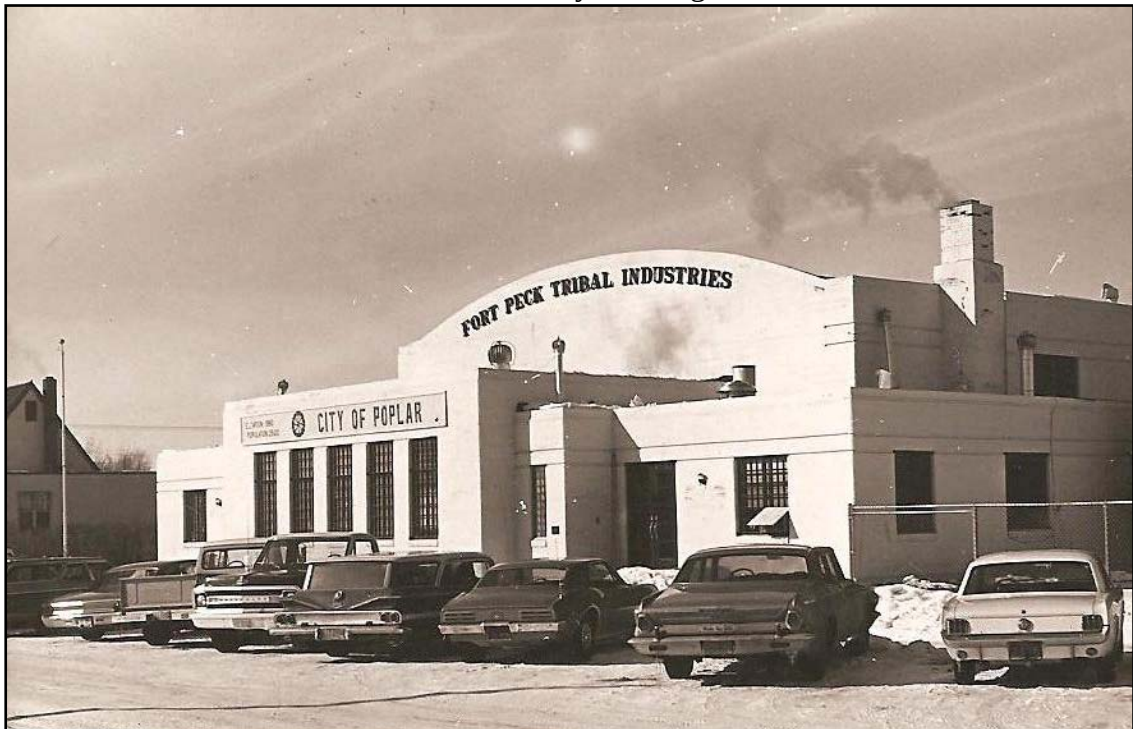
Figure 22. Fort Peck Tribal Industries, late 1960s or early 1970s (Poplar Shopper). FPTI was located in the New Deal era armory building.
