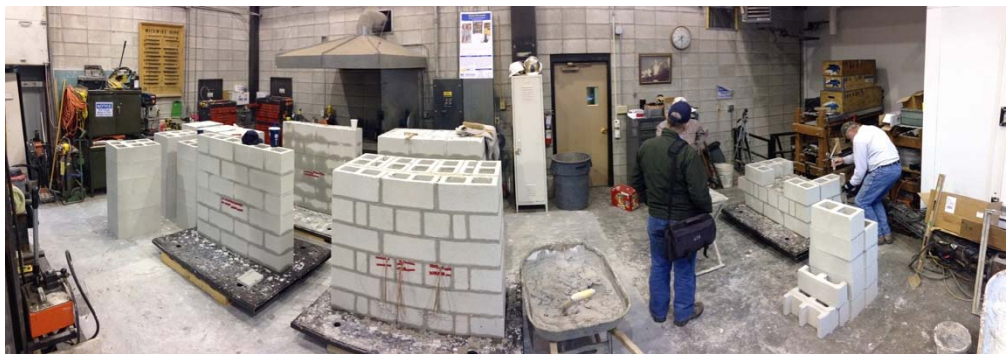
Figure 24. Wall specimens under construction
