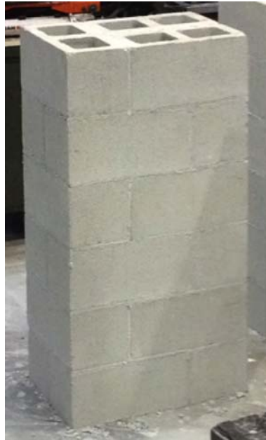
Figure 18. 6-course running bond layup prior to grouting
