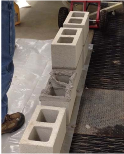
Figure 10. Construction of prisms
