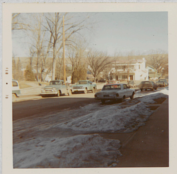
Fig. 16 East of Site
