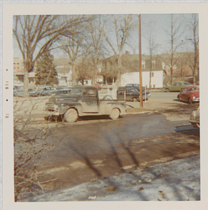
Fig. 15 East of Site
