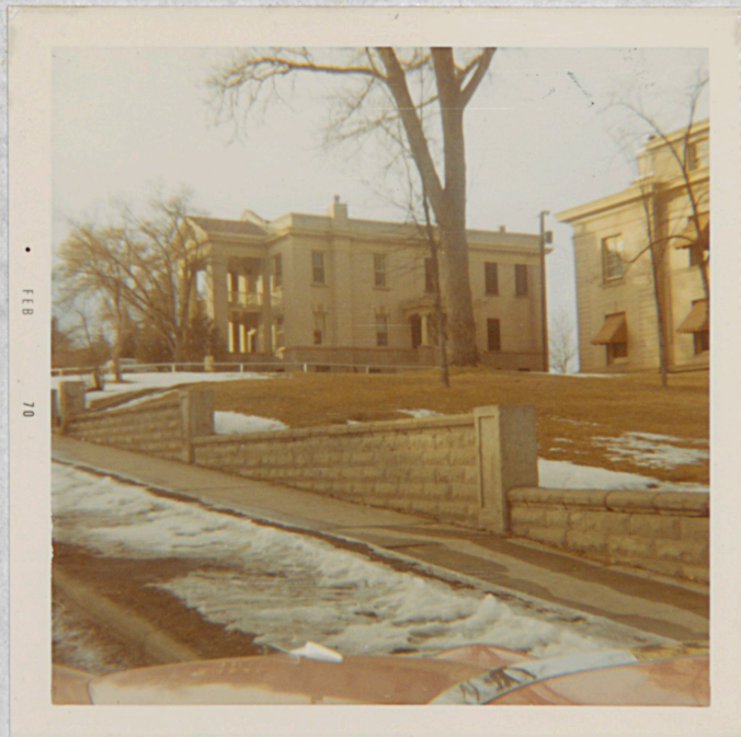
Fig. 7 Jail from East
