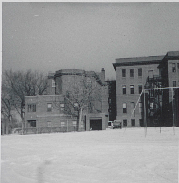
1. West Corner of South Elevation
