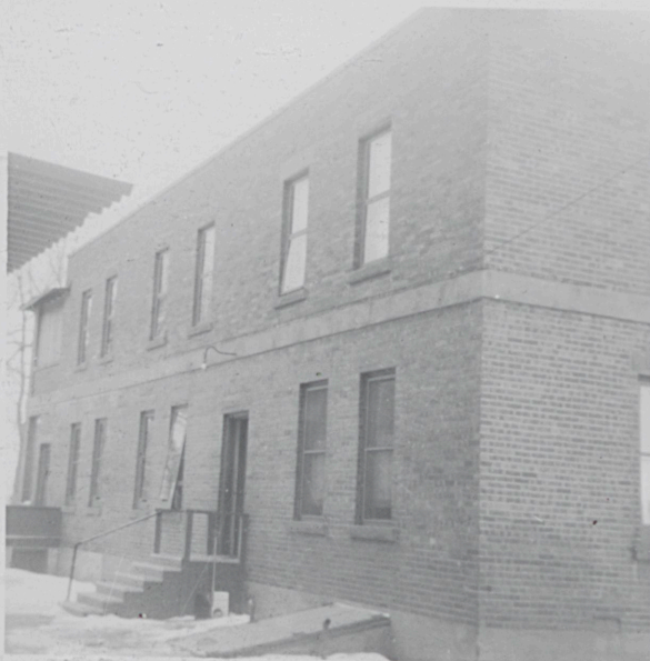
4. North Elevation of Little Boys's Building
