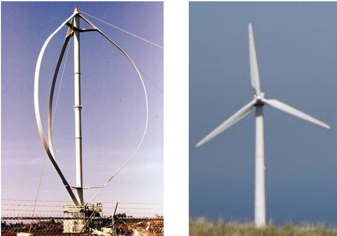
Figure 2: Wind turbines compared: a) Darrieus-type VAWT [16], b) HAWT [17]
