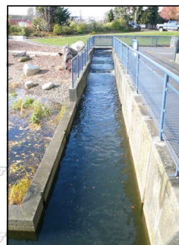
The fish ladder routes spawning salmon to holding pens. After enough salmon have congregated, they collect them and extract eggs and sperm.
