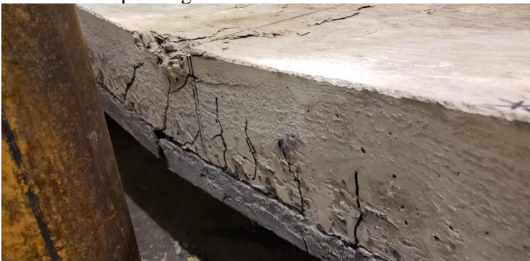
d) Midspan after failure, showing crushed concrete
