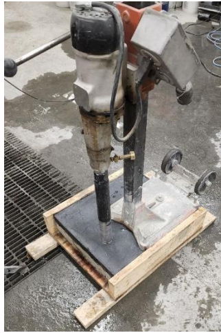
b) Core drill in place on slab
