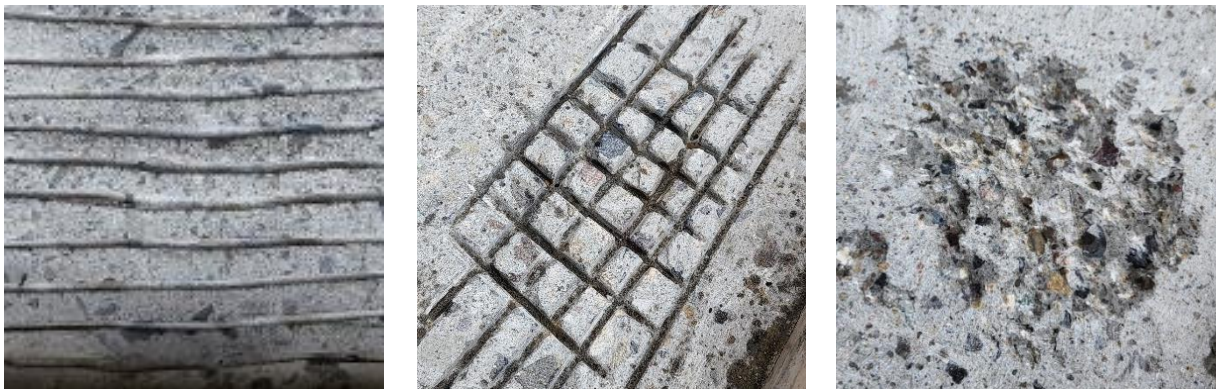
a) T Surface Preparation
