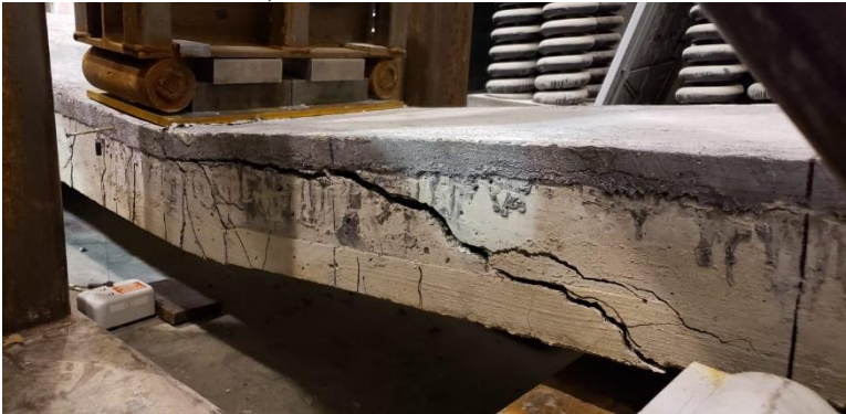
c) Crack widening/spreading at the end of testing
