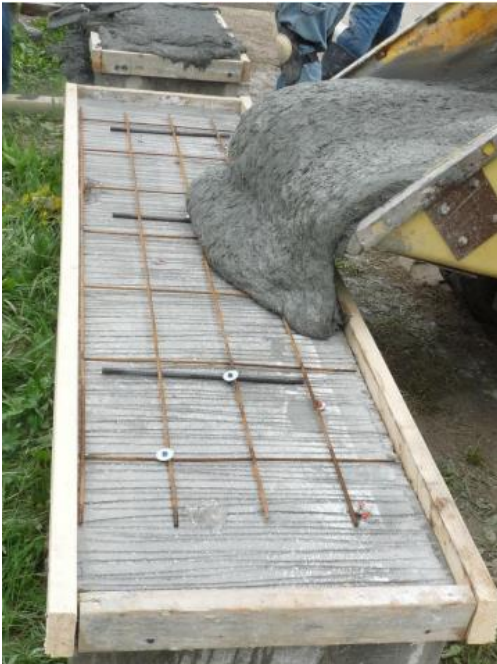
Figure 4: Casting UHPC on slab specimens [23]
