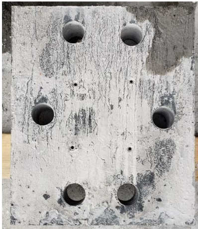
c) Slab after coring
