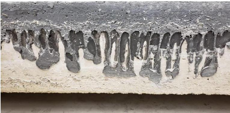
a) Before UHPC chipping
