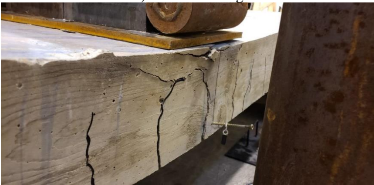
b) Concrete crushing prior to failing
