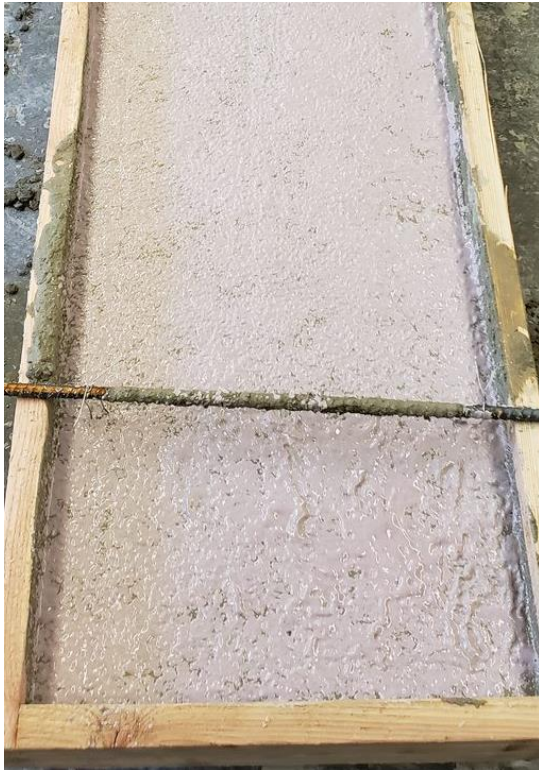
a) After surface retarder applied
