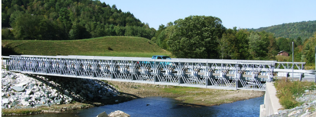
Figure 5. Acrow Bridge assembled using Several Layers of Panels to Achieve the Span (Acrow Corporation of America 2015)
