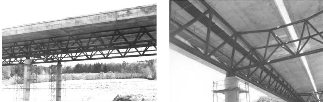
Figure 14. Lully Viaduct Space Truss (Dauner et al. 1998)
