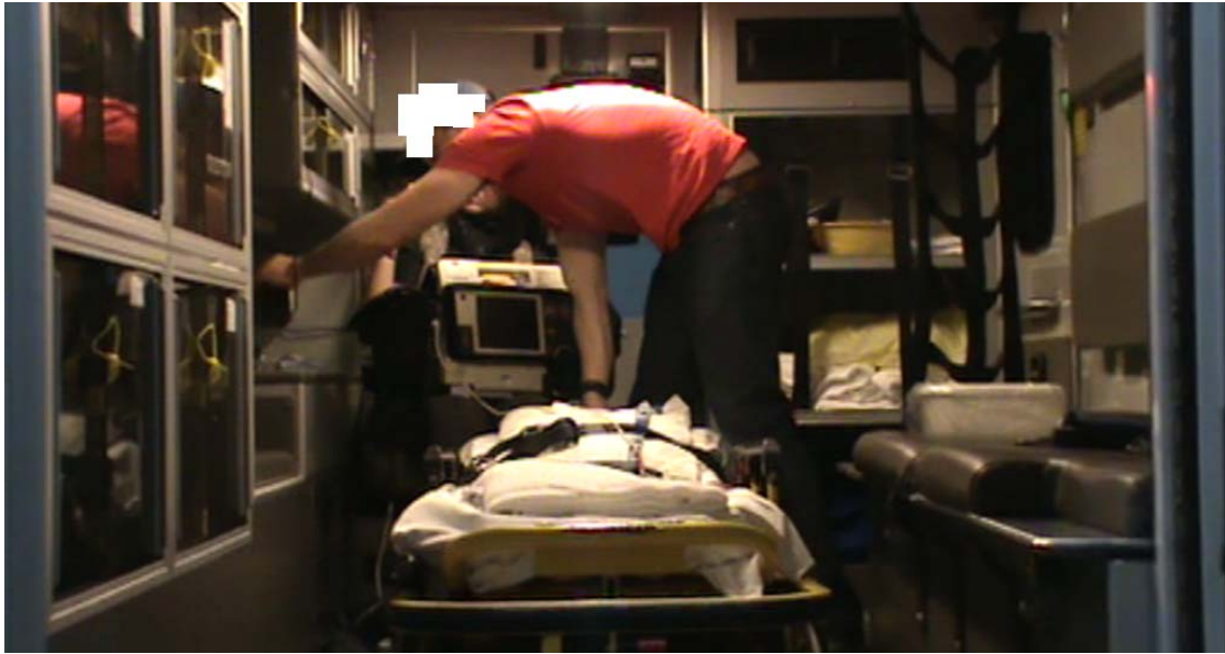
Figure 17. Reach from Bench Seat to Electrical Panel
